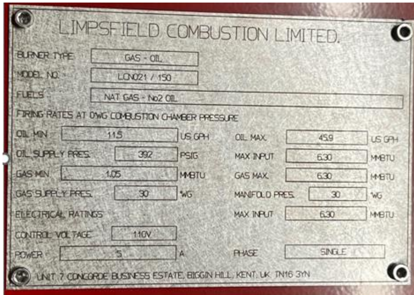
Spec Plate for Boiler #8
