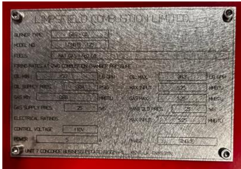
Spec Plate for Boiler #8
