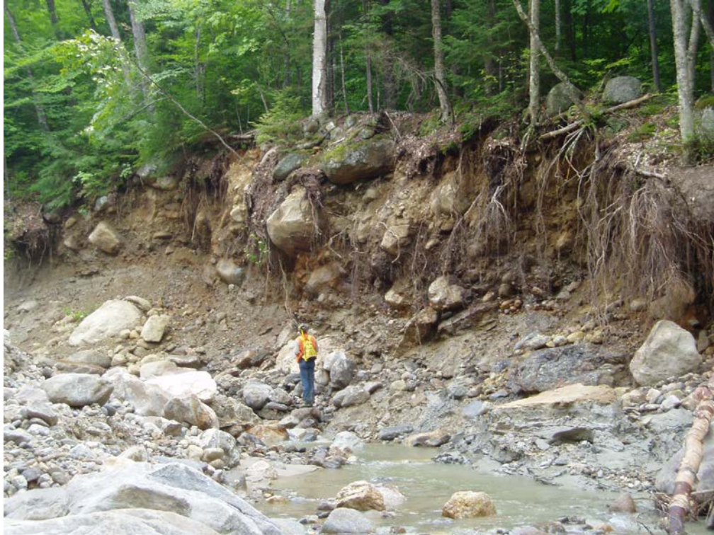
Bank erosion rated as Extreme.
