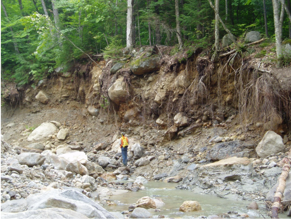
Photo 1: Photo taken in 2007 during storm damage assessment
