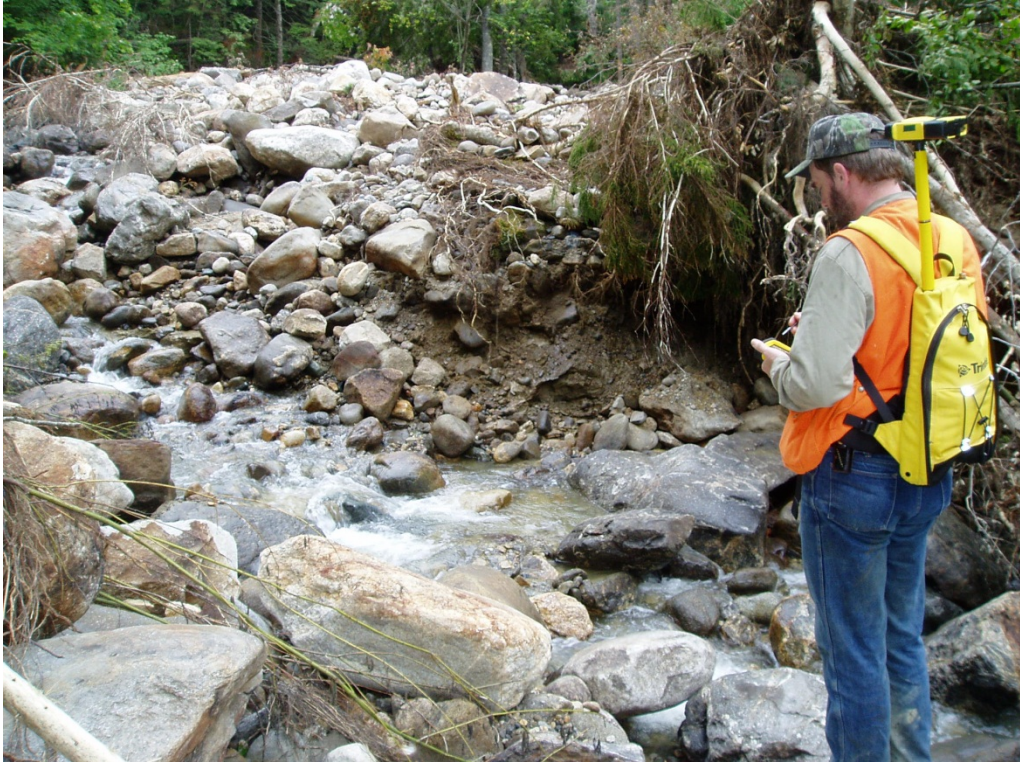
Photo 5: Photo taken in 2007 during storm damage assessment
